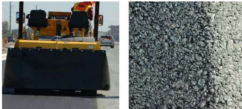
FIGURE 8. Tight longitudinal joints with no aggregate crushing
