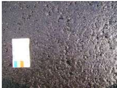
FIGURE22. Surface condition of the pavement (section 3)
