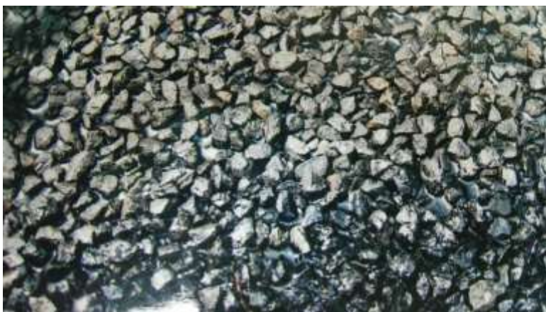
FIGURE27. Finished surface after compaction of VPT roller
