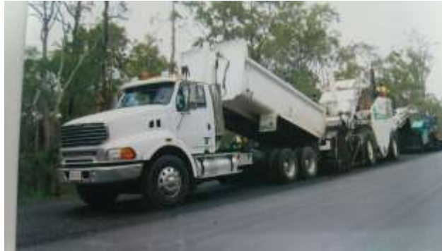
FIGURE24. Chip seal application
