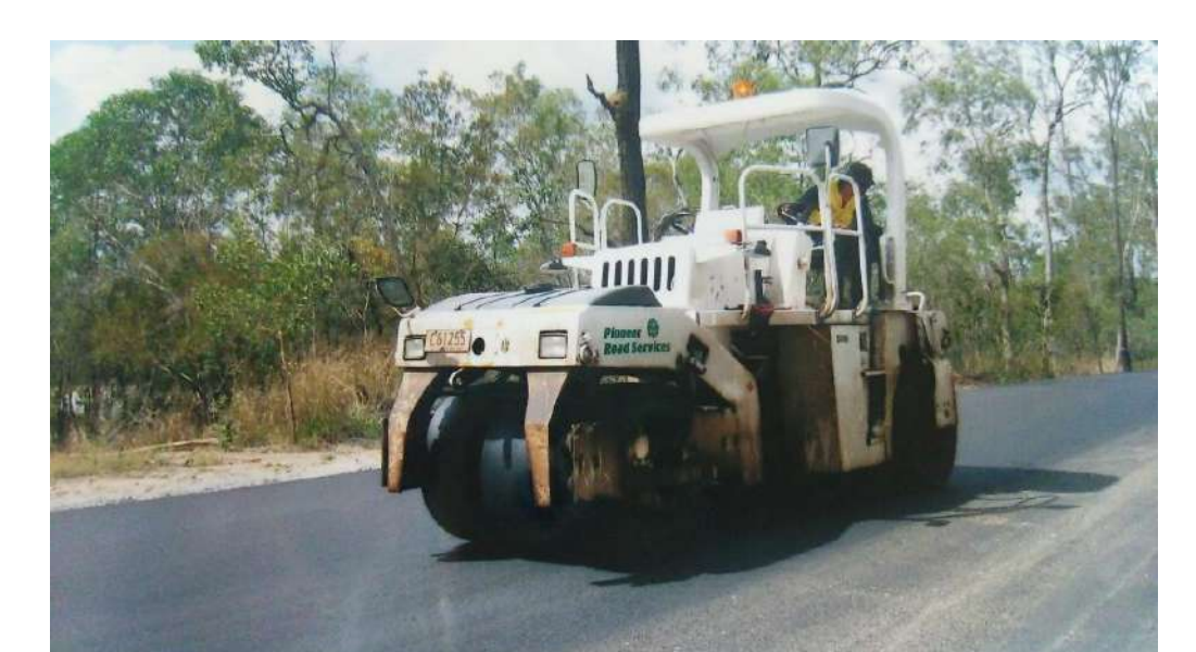
Compaction of Chip Seal Australia
