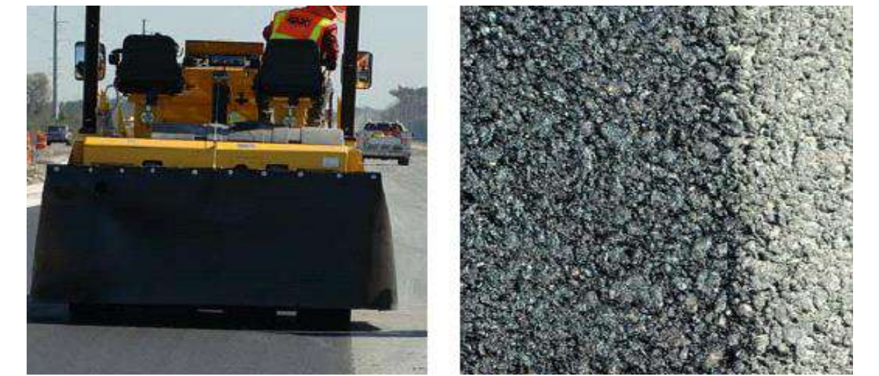
Tight longitudinal Joint
